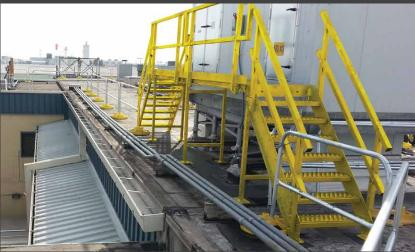
Crossover ladders can take on many shapes and sizes. From simple bridges to complex structures utilizing highly customized attachment and access points. All SRC Crossovers can come with a PE stamp ensuring structural integrity of the system. There is no limit to the types of crossover structures industry requires and almost no limit to the types of structures we can build.
