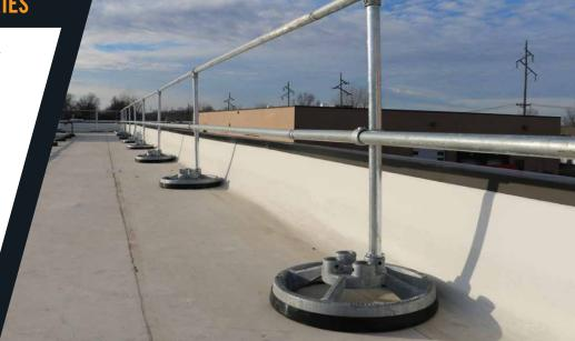
Rubber pads on the base plates act as a barrier between the base and sensitive roof surfaces.
